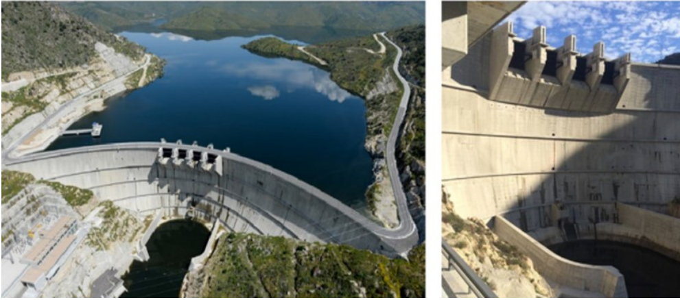
Figure 1: Baixo Sabor arch dam, reservoir and dam from above, and downstream spillway detail [21].
