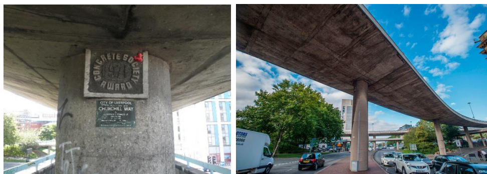
Figure 1: Churchill Way flyover, Liverpool, UK.
