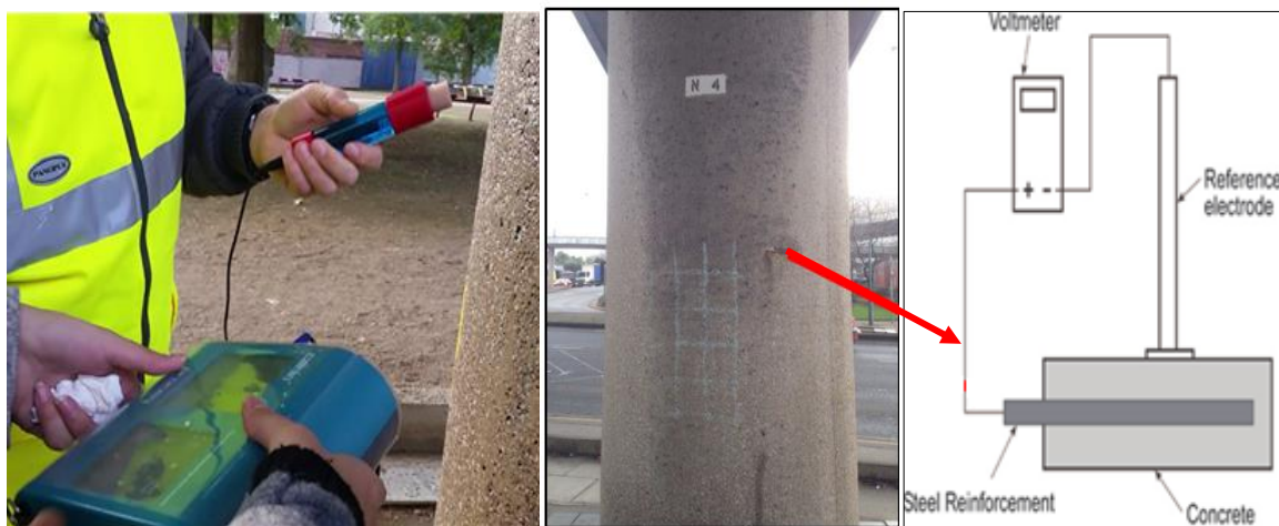
Figure 5: Conducting Half-cell corrosion potential testing.
